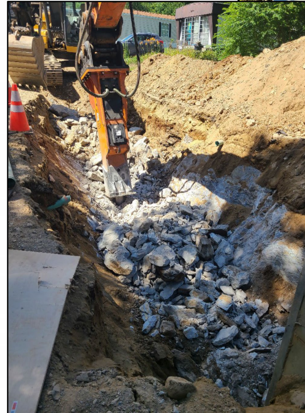
Ledge being hammered at project site
