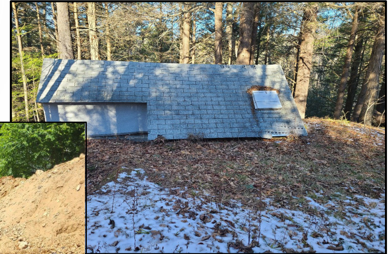
Abandoned wellhouse to be removed
